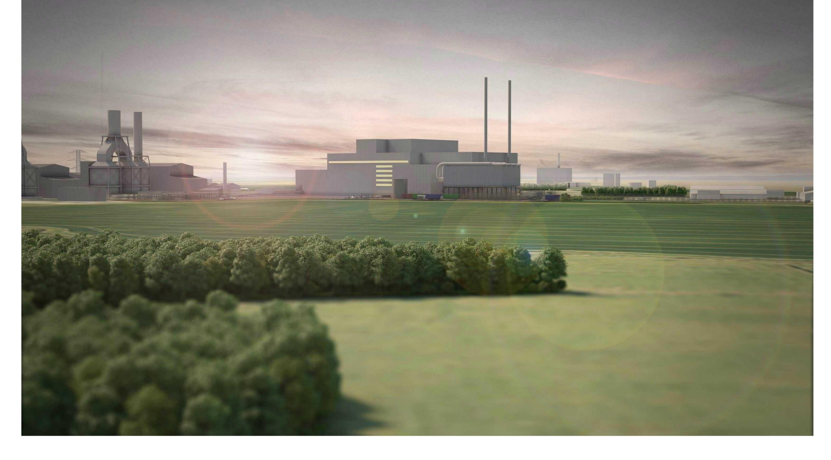
The stack height has been fixed at 102 m Above Ordnance Datum (approximately 100 m above the ground level).
