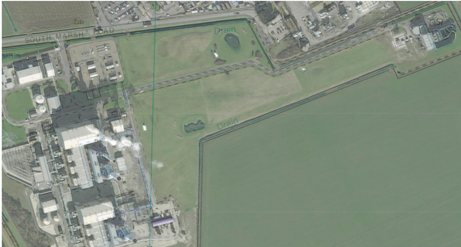
Plate 13B.3: Current aerial photograph of the Main Development Area ( https://historicensland.org.uk )
